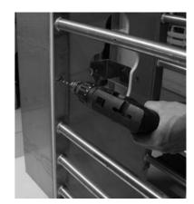
Fasten the antenna box to the side panel.
