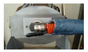
10. If a suction/pressure sensor is installed, install the isolation box as shown in the lower figures. Click the plastic tube into the isolation box (option) and install the heating cable above the sensor. The PG screw connection must points downwards.
